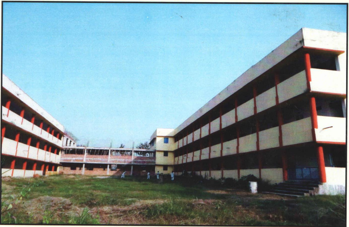
Building of Al-Habeeb Teacher's Training College Sector - VI, Bokaro Steel City - 827006 (Jharkhand)
